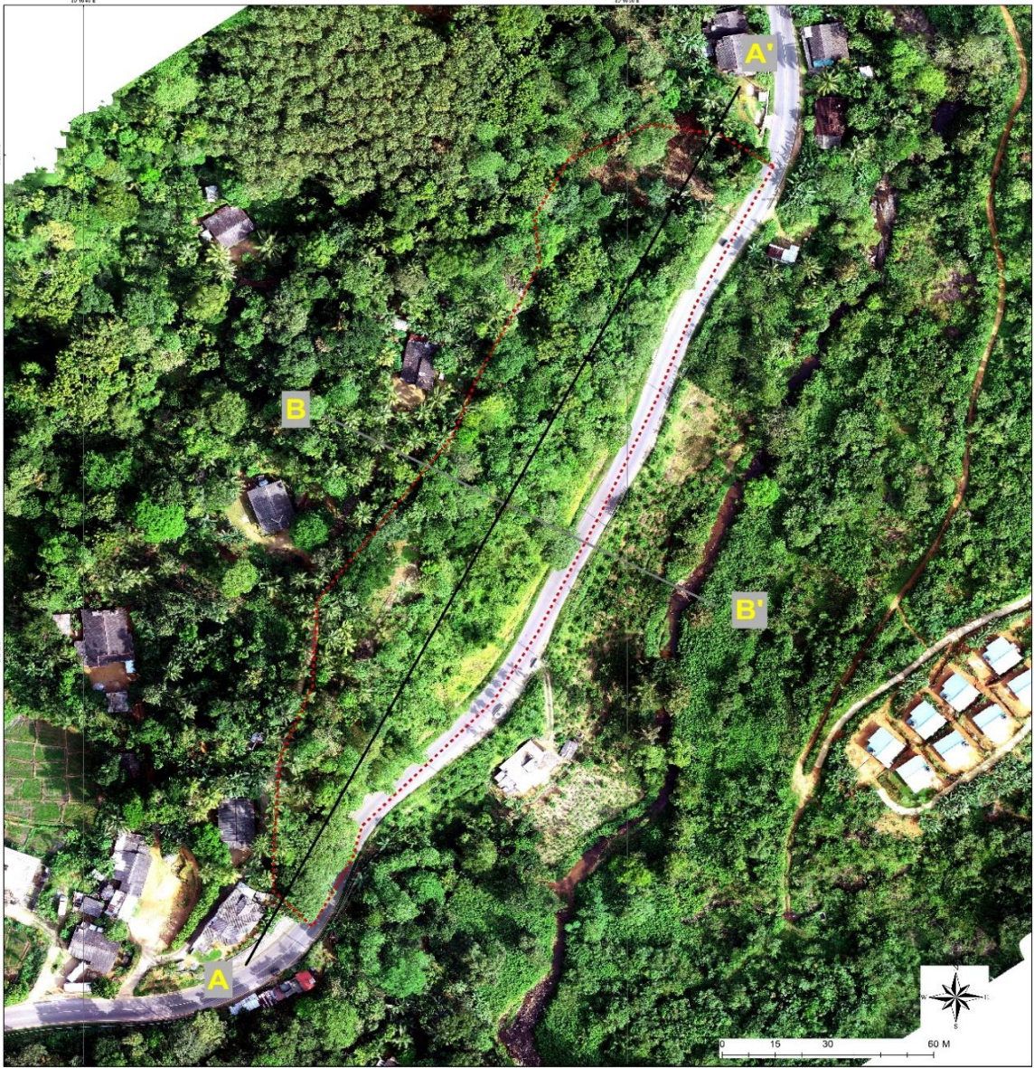
Landslide Mitigation Site No - 122 - Kegalle- Dehiovita- B-110- Eheliyagoda-Dehiovita road. Culvert no. 5/6 - (AIIB Project)
